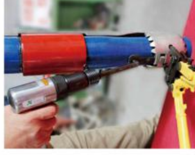
气动冲击枪油管安装 Install pneumatic impact gun hose tubing
