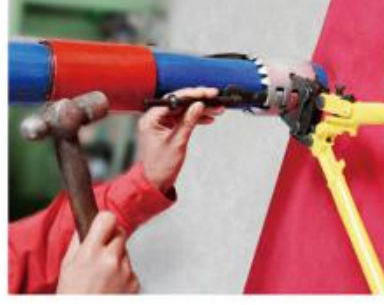
手动油管安装 Manual pipe installation
